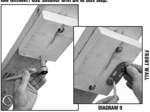
Mount **2"** x **6"** x 7" riser board on front mounting board centered between the two Pigtail Lag Screws (B). Drill <sup>5</sup>/32" (4 mm) holes. Attach riser boards using two <sup>1</sup>/4" (6 mm) Lag Bolts (I) and Washers (J) (included). Do not over-tighten.
